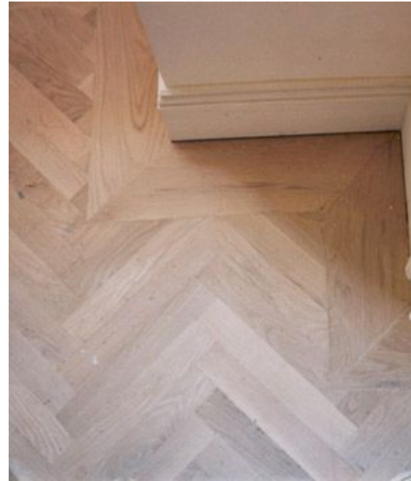
Chevron Wood flooring with border detail in all but shower and elevated bath area
